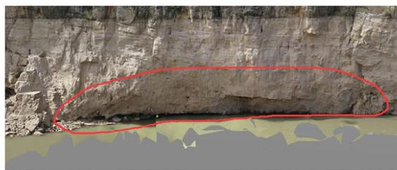
(f) Rock block B5 is compressed and falling to form a cavity.
